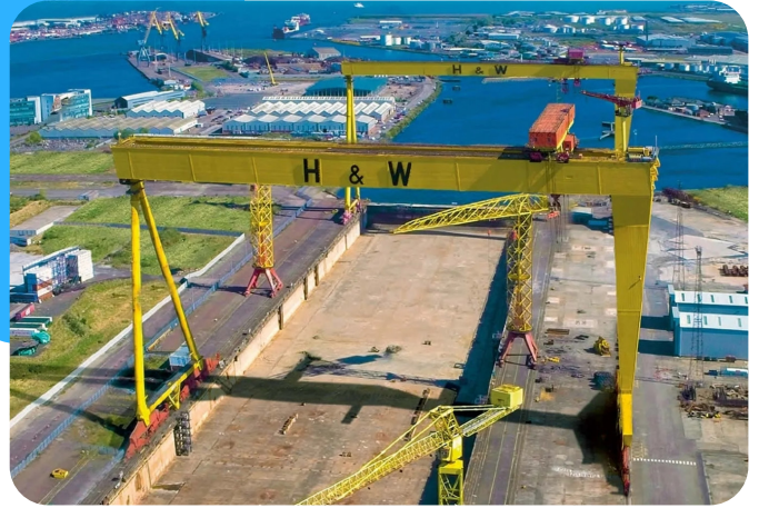
Panoramic Harland & Wolff overhead cranes
