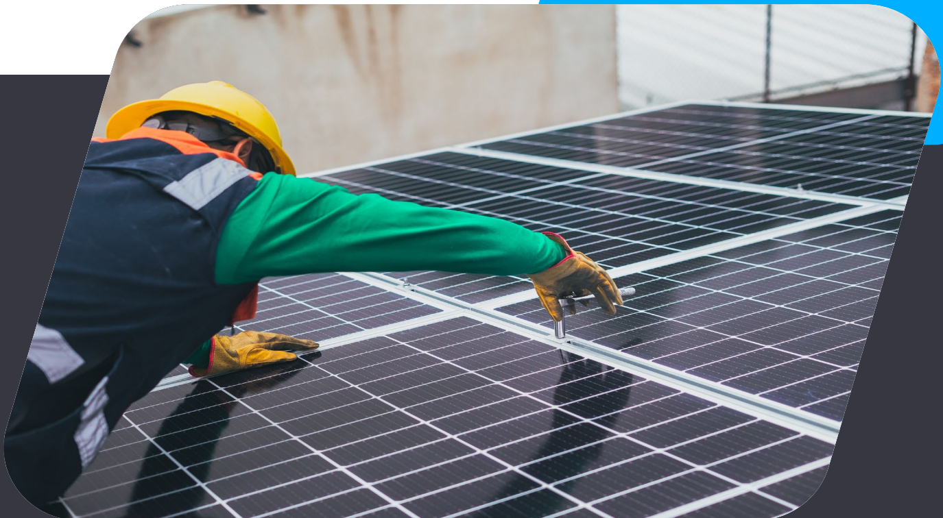
Installation Solar Panel
